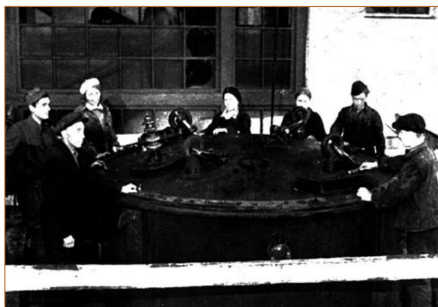
Reconstruction of the Volkhov hydroelectric station after bombing.1943
