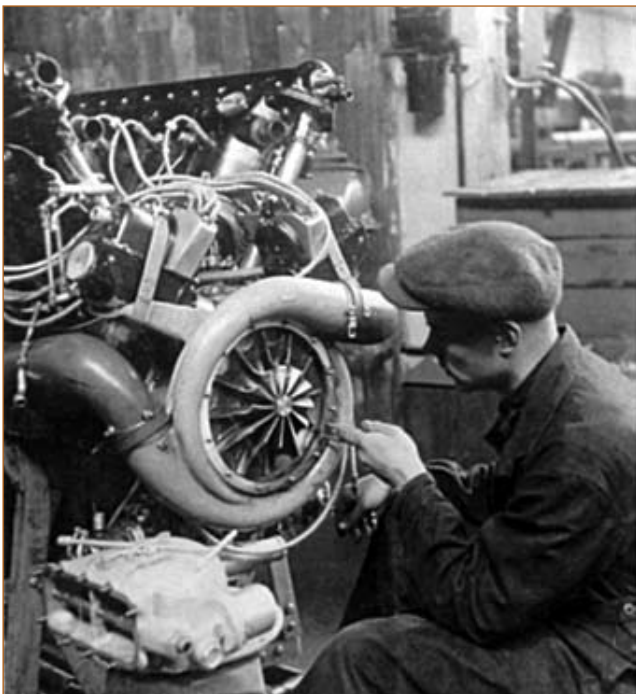
The aircraft engine M-105 PF assembly. Ufa Engine Plant №26. 1944
